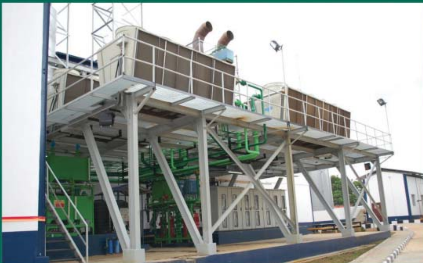
The 10MW Alausa Independent Power Project funded by Fidelity was commissioned in October 2013. The project was the 3rd Partnership between Lagos State and the Bank in the area of IPPs.
