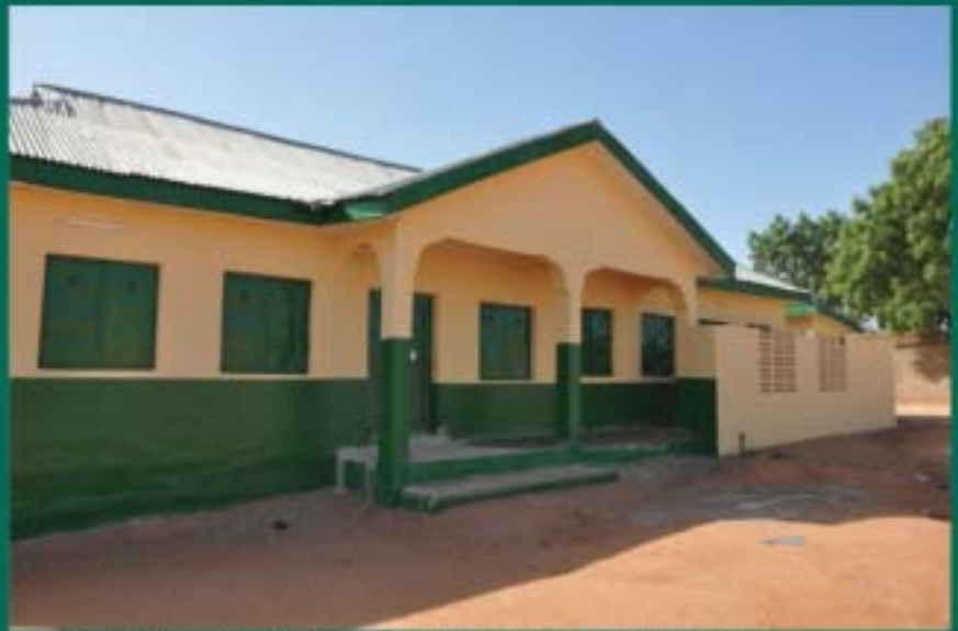
One of the classroom blocks renovated at Gombe Special School
