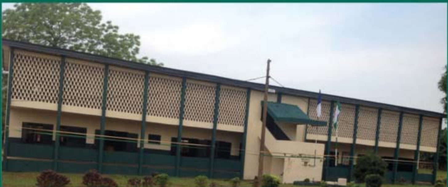
Classroom block renovated for Our Lady's High School, Onitsha.
